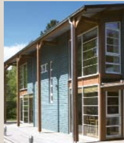
Raising a frame (top); Inchdryne Lodge (above); an open-plan living space (opposite, top) and an isolated study retreat (opposite, bottom).
