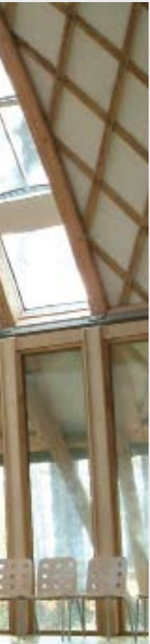
Glulam beams supporting the roof of the debating chamber in the Scottish Parliament building (above).
