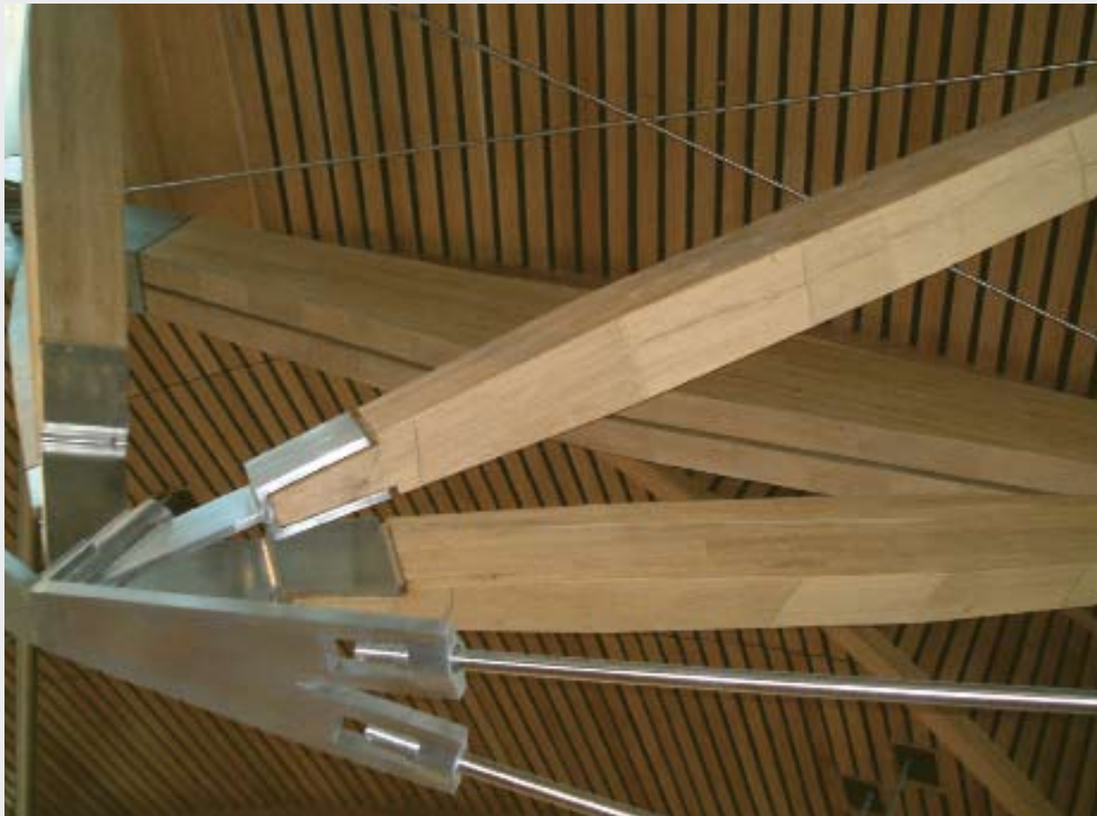
Glulam beams supporting the roof of the debating chamber in the Scottish Parliament building (above).
